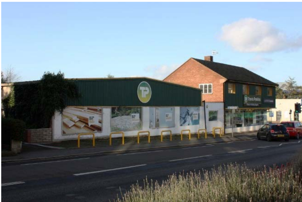
Plate 27: Buildings on the west side of Boythorpe Road
