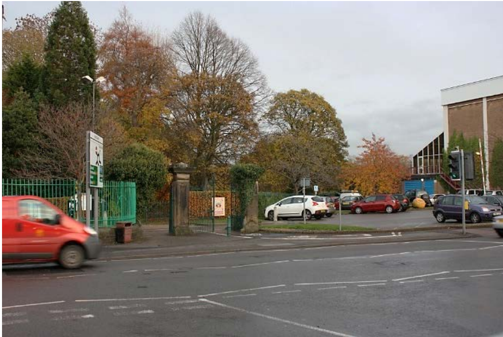
Plate 26: The original main entrance to the park from Boythorpe Road and an adjacent parking area
