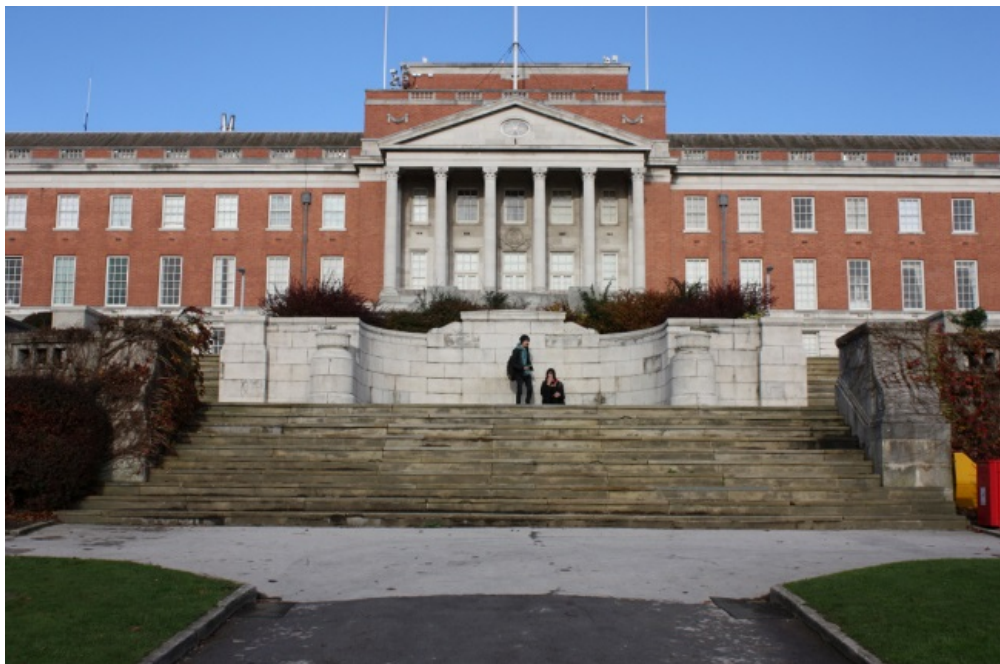
Plate 15: Chesterfield Town Hall with the war memorial and steps in front
