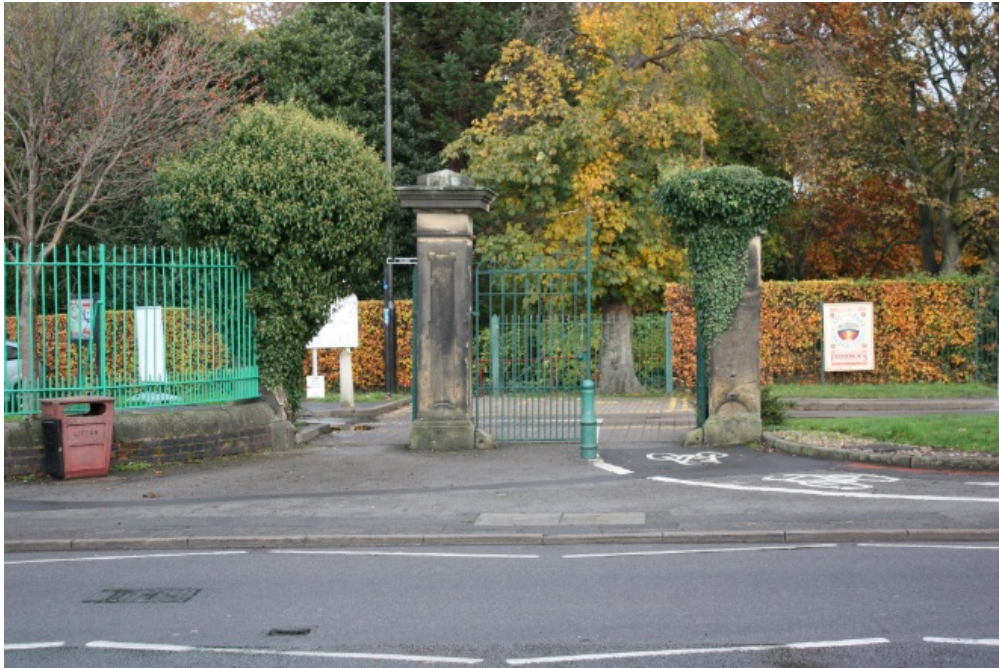
Plate 8: The west entrance from Boythorpe Road
