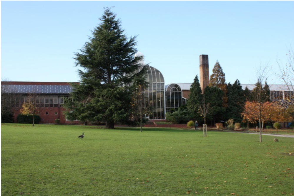
Plate 24: The east-facing park façade of the sports centre
