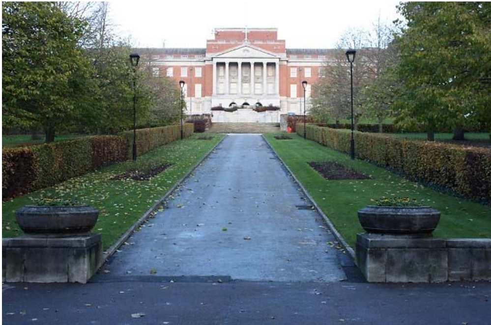
Plate 16: Chesterfield Town Hall with the war memorial and steps in front, seen from the approach through the Shentall Gardens
